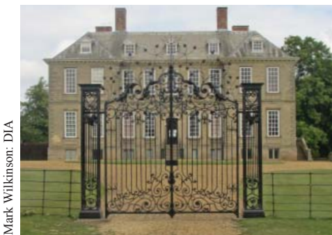
Iron gates after restoration
