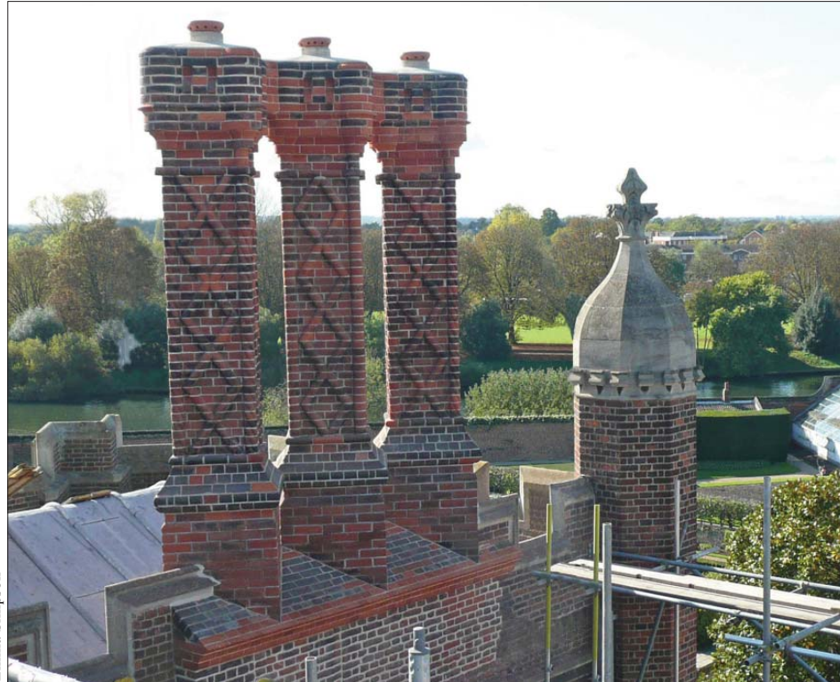
The three chimney stacks after strengthening and repair
