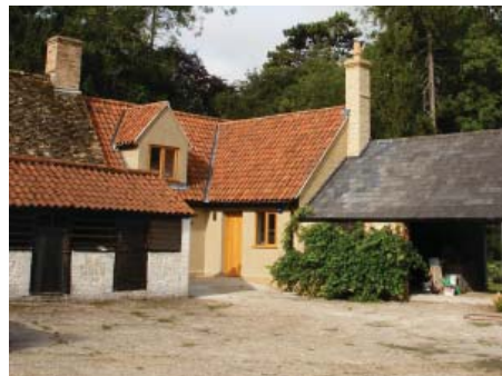
New extension replacing a former cowshed
