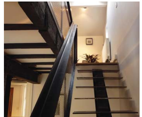
New steel stair leading to the upper studio
