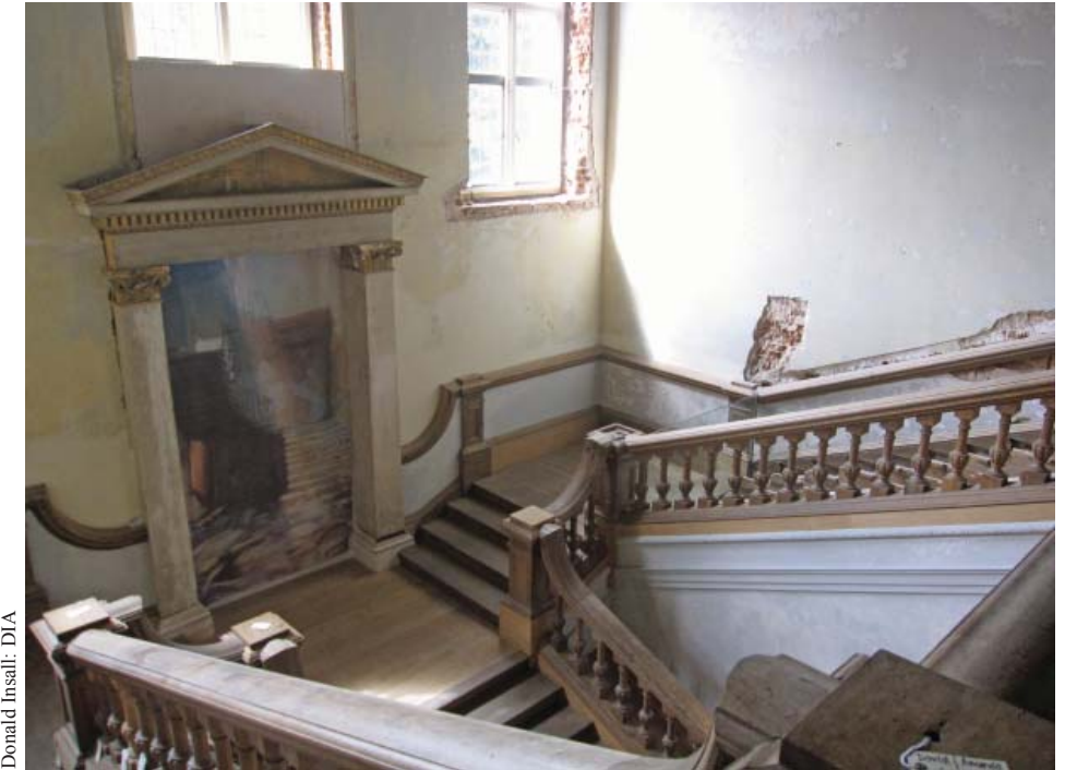
The Grange staircase and door surround reinstated after almost 40 years
