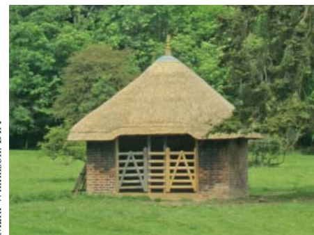
The reinstated thatched roof on the Deer Shelter
