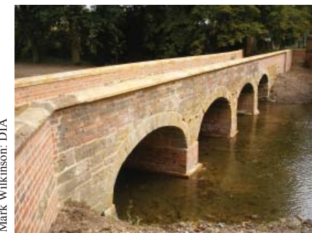
Completed repairs to the Charles I Bridge
