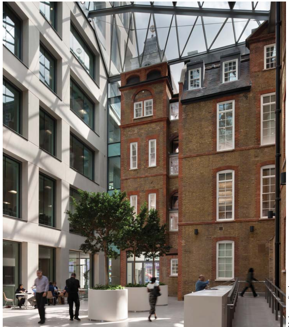
Glass-roofed atrium of the Unison Centre unites the old with the new
