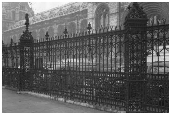
Waterhouse Building: Railing at the main entrance on Cromwell Road in 1951
