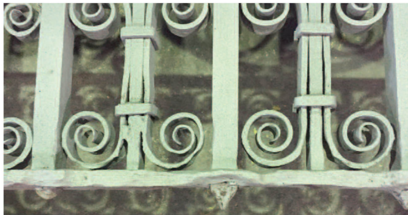
Above: Typical corrosion of bottom scrollwork. Right: photographs showing the railings after the completion of the Natural History Museum project earlier this year
