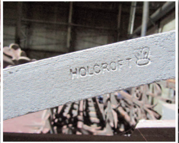
Main picture: the Natural History Museum railing after the completion of the project. Above: One of a number of iron-maker's stamps. Top: an advertisement from the Portfield Ironworks – makers of at least some of the wrought iron
